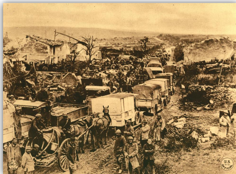
Congestion and muddy roads around Esnes made transportation difficult
